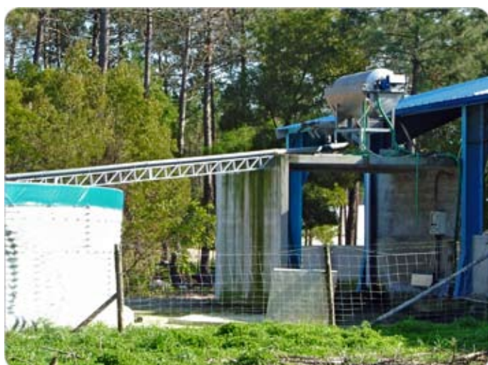
Sewage Treatment Station
